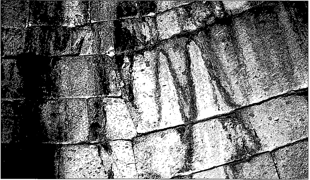
Fig. 11. The left side inclination of the huge lintelblock in the Atreus tomb (seen from the inside of the burial chamber) which was used to move the block on the plain. Photograph R. Santillo.
