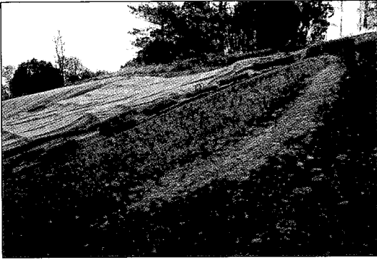
Fig. 3. Cement barrier that conducts away the water from rock-carvings at Aspeberget, Tanum. Photo: Håkan Karlsson.
