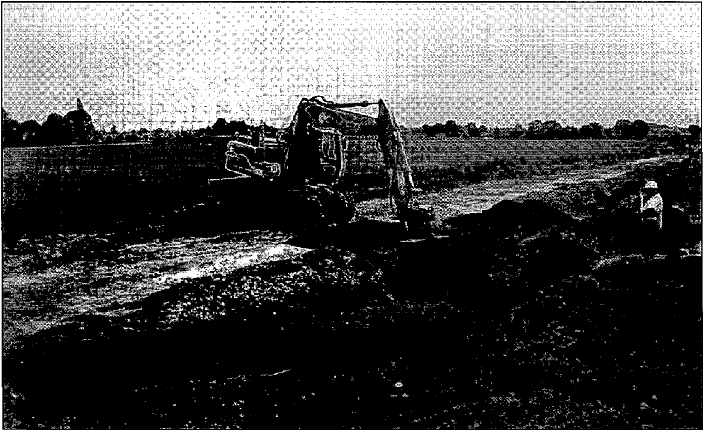
Fig. 2. Removing topsoil in Burlöv, Malmö. Photo: Ulf Celin.
