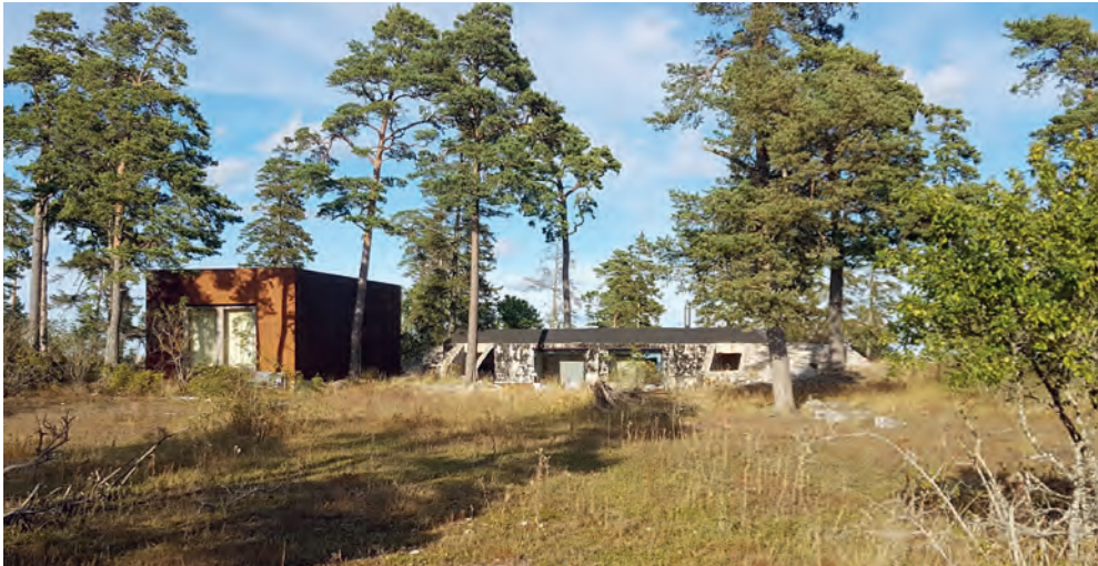
6. A desirable original bunker, redesigned into an exclusive holiday home, supplemented with a housing cube in trendy corten steel. Photo: M. Frihammar.
