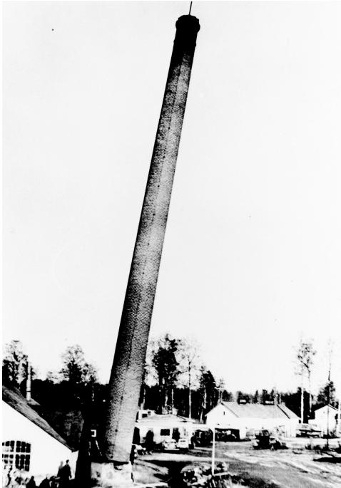
Demolishing the smokestack in 1966. Photo: The Archive of Traditional Society of Ähtäri.
