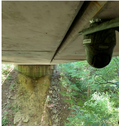
Figure 1. A trail camera deployed underneath a bridge
