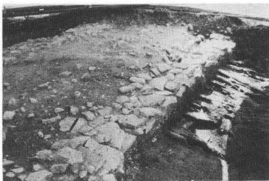
Photo 4. A 3.5 m wide stone foundation laying on a wooden supporting structure.
