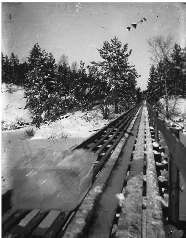
Image 3. An ice chute with a block of ice in motion, at Hellefjorden in the Kragerø district, ca. 1910. Photographer: Johan Lyng Olsen, Berg Kragerø Museum/Telemark Museum Collections, BKM.F.000845.
