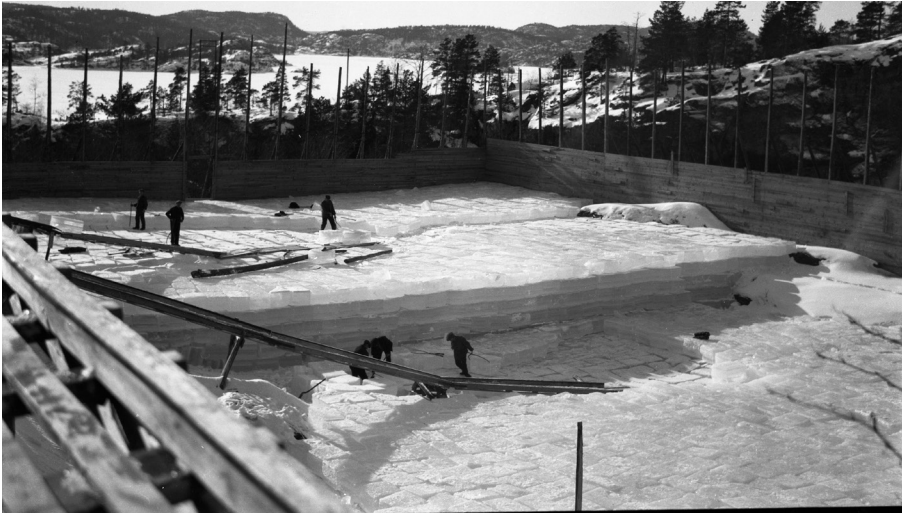
Image 4. Thousands of tons of ice stacked in a roofless stack, awaiting transportation. From Svartjern, Kragerø, date and photographer unknown (probably after 1900). Berg Kragerø Museum/Telemark Museum Collections, BKM.F.003905.
