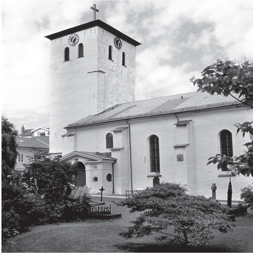
Figure 5. Mariakyrkan in Marstrand, facing northwest. The remains of the Franciscan friary partially excavated between 2017 and 2018 are located in the cemetery area on the left hand side of the photograph. Photo: Tomas Brandt, Bohusläns museum.
