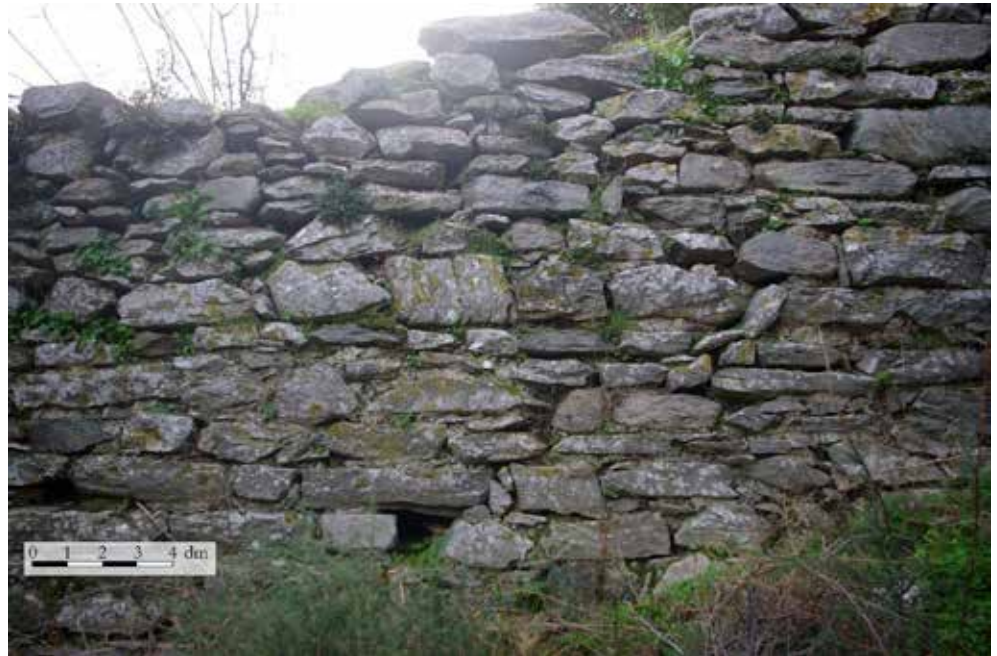
Fig. 4. Late wall, outer face, in mortared rubble masonry. Photograph by Patrik Klingborg.
