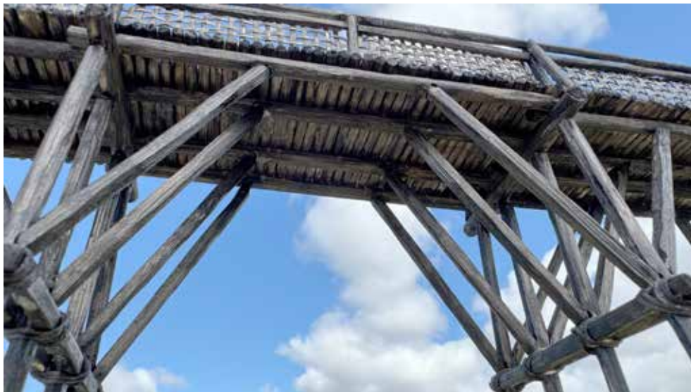
Fig. 1. The Spina bridge, miniature model reconstruction in wood (model by R. Holmgren). Copyright: Richard Holmgren ARCDIOC.
