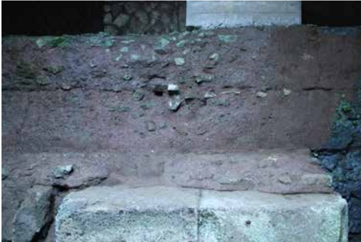
Fig. 7a (above, left). Concrete foundation wall m , east section, partly overlaying ashlar foundation wall F x . View from the west. Photograph by Henrik Gerding.
