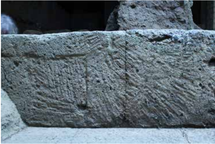
Fig. 11a (above, left). Detail of ashlar blocks in foundation wall F_2 . View from the north. Photograph by Henrik Gerding.
