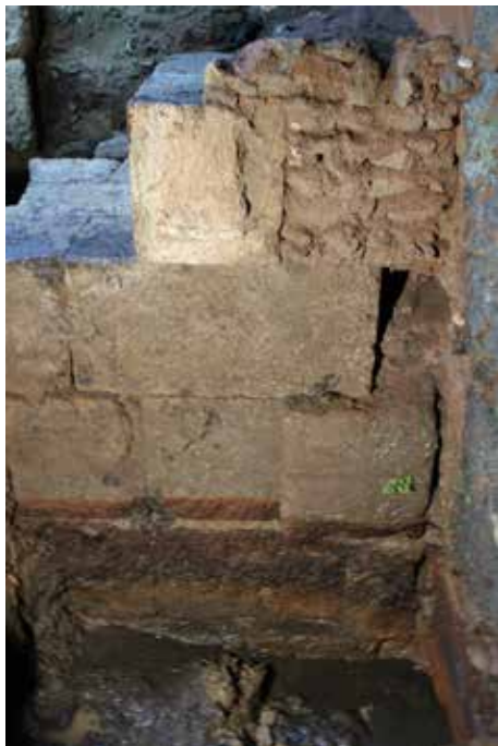
Fig. 10a (above, left). South side of ashlar foundation wall F_2 . View from the south. Note that a fifth course of blocks is visible at the bottom. The block furthest to the right in the fourth course has been cut to accommodate the foundation trench for concrete foundation wall m . Photograph by Henrik Gerding.
