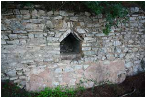
Fig. 2b. House-shaped feature in the aqueduct. Note the pink plaster covering the aqueduct. Photograph by Patrik Klingborg.
