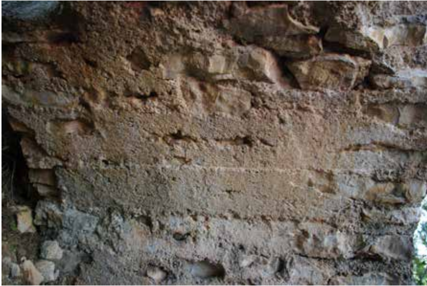
Fig. 2d. Imprints in the mortar of wooden moulds from the construction of the first arch from the west. Photograph by Patrik Klingborg.
