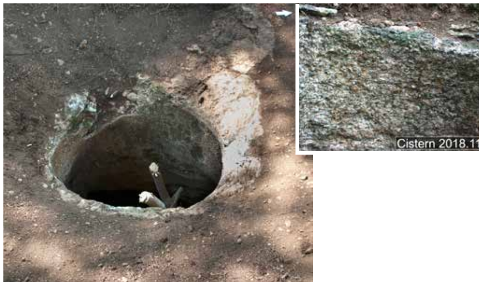
Fig. 14. Cistern 2018.11 , mouth, with a diameter of 85–90 cm. With detail of lining. Photographs by Patrik Klingborg.
