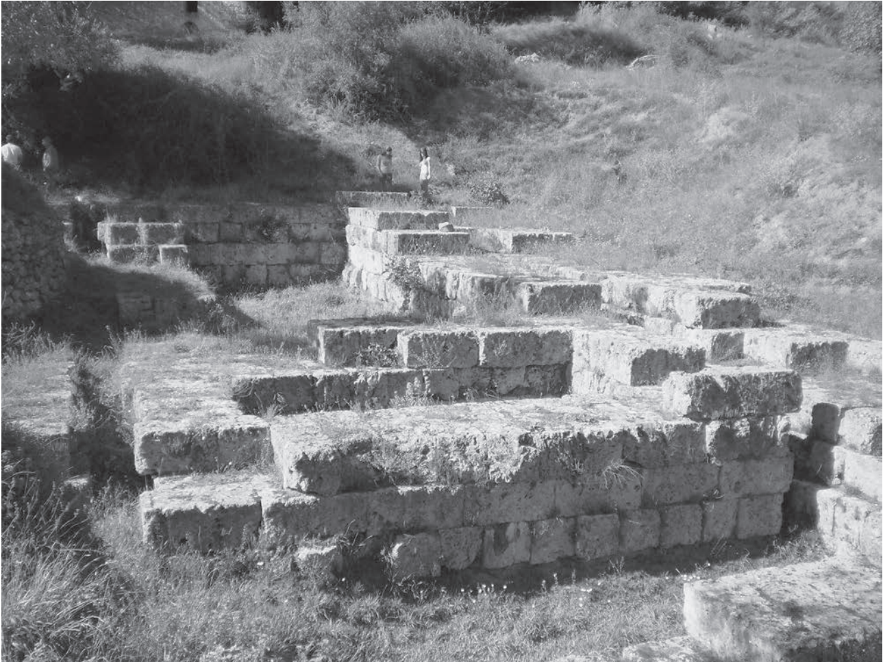
Fig. 6. The construction of the foundation of the Temple of Asclepius as seen from SE, in November 2015. Photo by C. Kanellopoulos.
