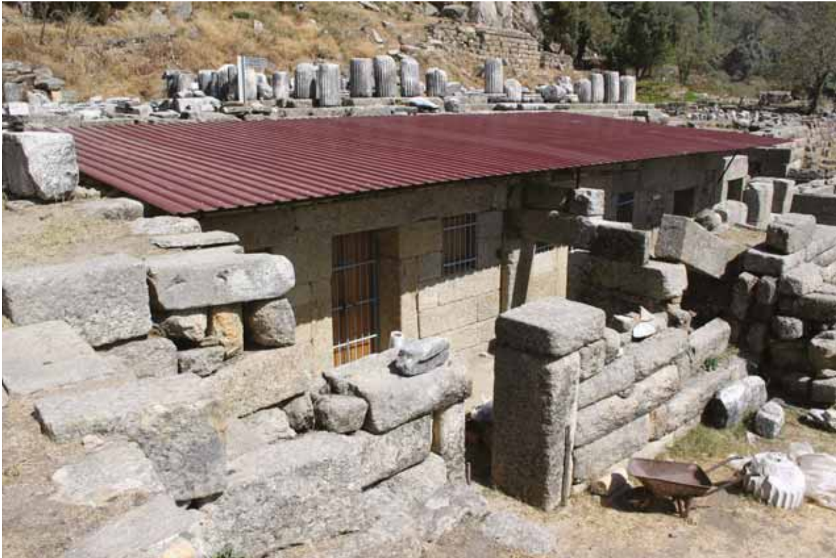
Fig. 33. The new metal roof over the storage rooms.
