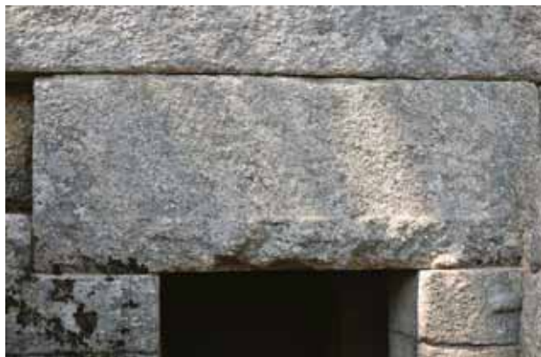
Fig. 44. The lintel above the doorway of the antechamber, with vertical dowel cuts on both sides.
