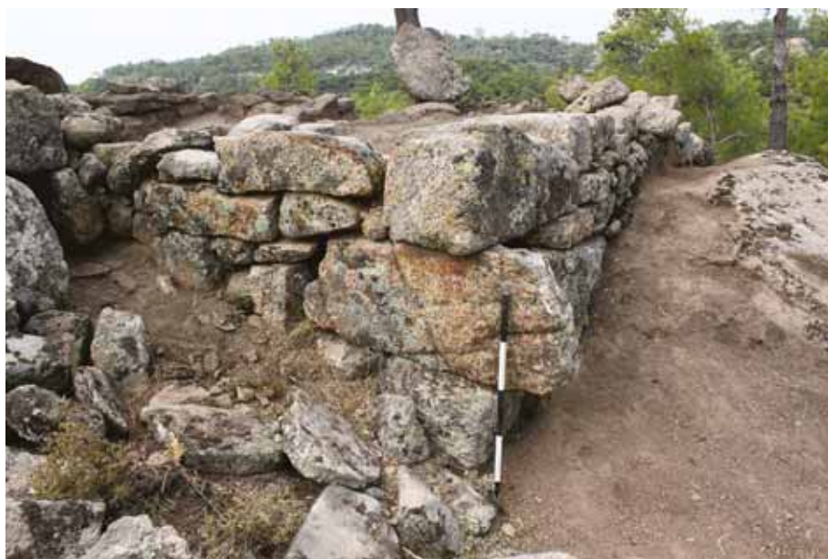
Fig. 4. Plated corner blocks in the tower's northeast corner.
