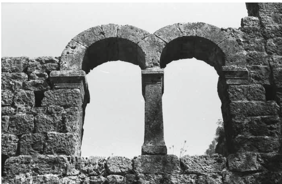
Fig. 15. The large building: the window.
