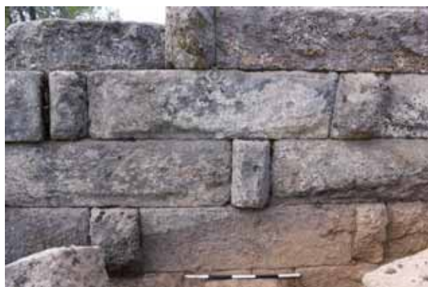
Fig. 6. Hekatomnid header-and-stretcher masonry of the central tower.
