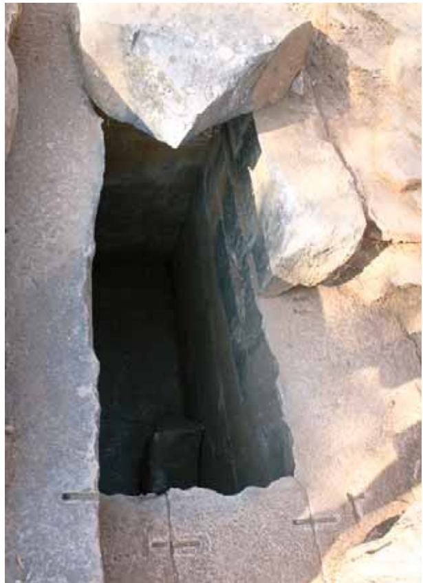
Fig. 86. Pi-shaped clamps on the top of the north wall of the main chamber.
