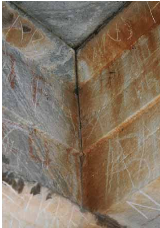
Fig. 90. Detail of the corner between a ceiling beam and the epikranitis of the wall in the chamber.
