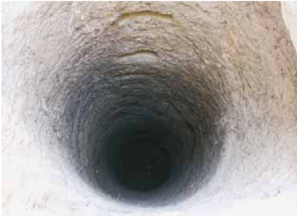
Fig. 23. View into the well, excavated to a depth of 6.7 m.
