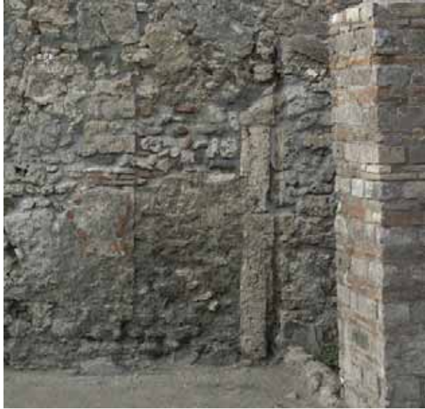
Fig. 38. Detail of Fig. 37: walled-up north doorway of the atrium area of V 1,23, the north House of Caecilius Iucundus. Note the clay lining half way up in the doorway fill and its relation to the plaster (full of pottery sherds) of the north wall proper. By Hans Thorvid.
