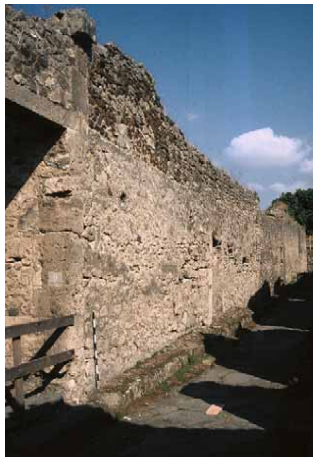
Fig. 4. Vicolo di Caecilius Lucundus looking north. The posticum of the Casa del Torello in the foreground. The façades display original rubble masonry. The dark lava incertum of the North House of Caecilius Lucundus is easily recognised in between the light masonry used for the façades of the South House and the Casa degli Epigrammi greci. By Arja Karivieri.
