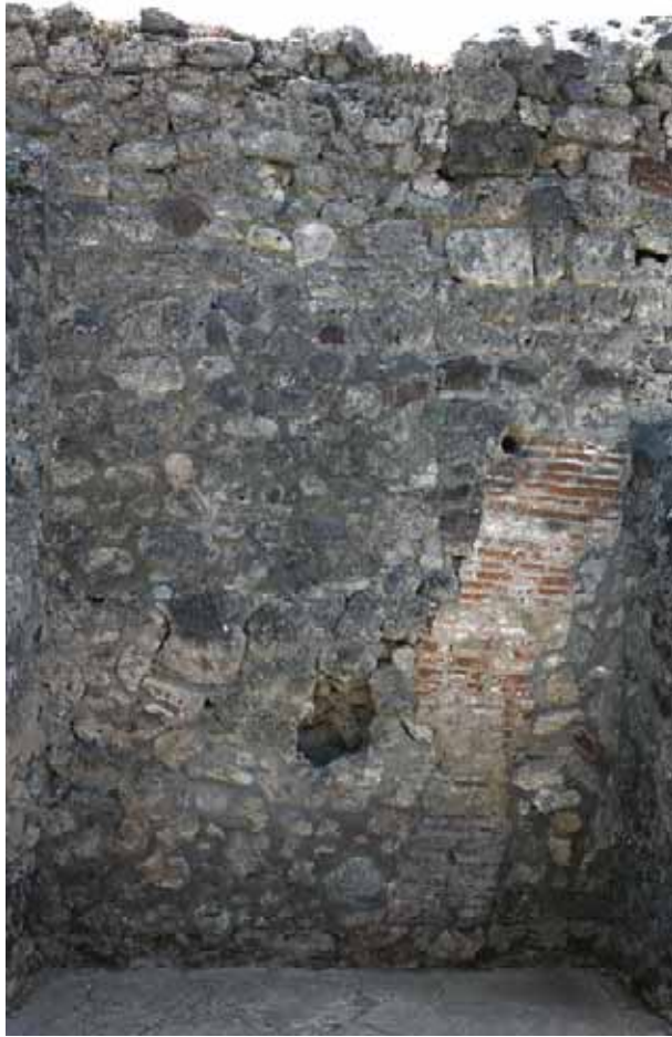
Fig. 23. Brick stitch repairing a fissure in the facing of the south wall belonging to the rear shop (b) of taberna V 1 , 24. By Hans Thörvid.
