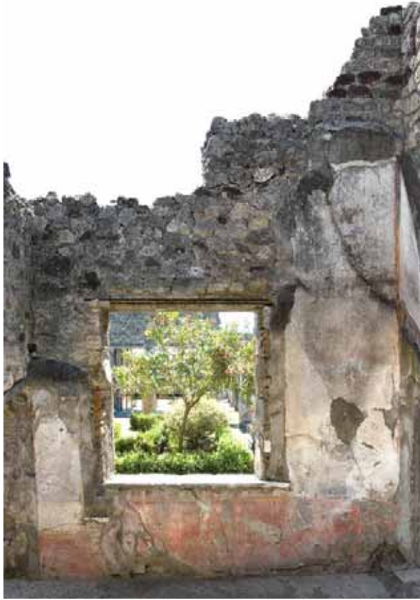
Fig. 26. Window with garden view. West wall of room s of the South House of Caecilius Iucundus. Note the sunken S part of the wall and the broken window-sill. By Hans Thörnd.
