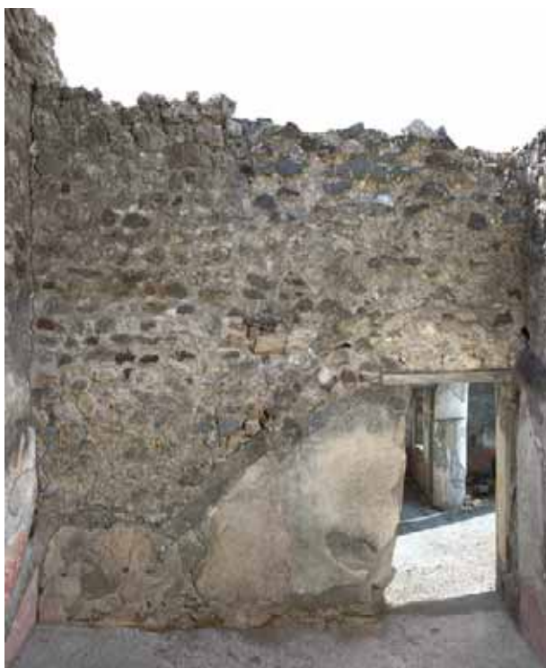
Fig. 25. The South House of Caecilius Iucundus, south wall of the garden room s . Note the collapsed state of the wall, partly sunken into the cellar beneath. By Hans Thorvid.
