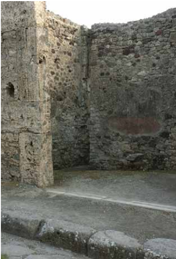
Fig. 22. Northeast corner of taberna V 1,25. Note the drain of a second-storey latrine and the position of the cesspit, corresponding on the other side of the boundary wall to that of the storage pit in taberna V 1, 24a. The southern part of the staircase base is original. By Hans Thornvid.
