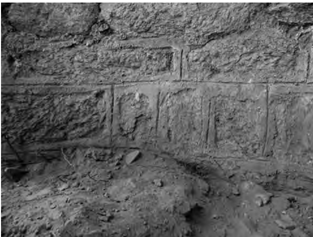
Fig. 37. Patterns of ashlar masonry drawn in the preserved mortar in the north apse.
